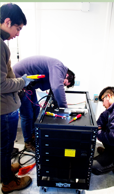
Installing the UPS.
